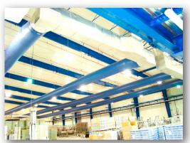
DuctSox products were initially developed exclusively for use in the foo processing industry. The flexible fabric is a cost effective alternative to insulated stainless steel ducting and diffusers. Draft-free airflow through the woven fabric improves comfort for employees and reduces dehydration in the end product.
